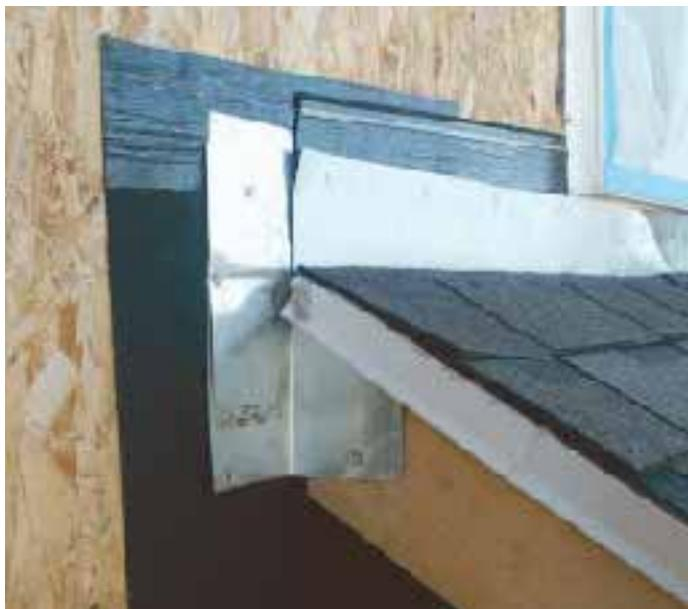
Here, the window installers and the roofers have not coordinated their work. Roof flashing will effectively catch water coming off the main wall if stucco papers are applied to lap over it. However, the window flange dumps behind the roof flashing instead of onto it. The author's crew removed this window and reflashed the opening before reinstalling the window.
